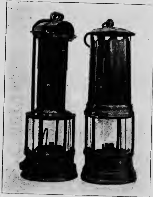
FIG. IV.—Clanny Lamps.
